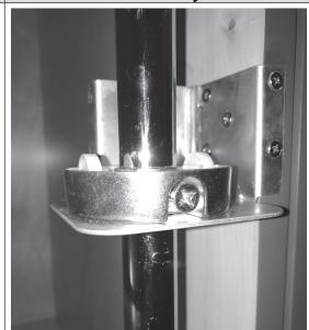
Slide the Upper Hub Assembly onto the pole and position the bottom of the bracket on the line drawn previously. Firmly secure with five #8 X 5/8" Flat Head Phillis Wood screws provided.
