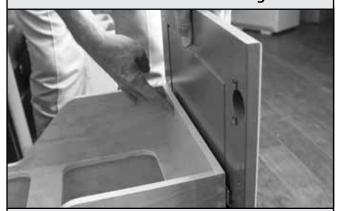
Adjust door-mounting brackets out to the desired location. Attach 1 square of double-sided foam tape to each door bracket. Close the organizer, visually line up the door and press door firmly against the organizer so that door sticks to tape on brackets. Open organizer and secure brackets with provided #6 x 1/2" screws
