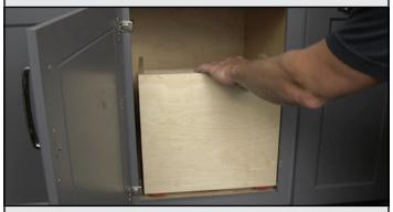
Place the trash organizer onto the undermount slides. Push the unit into the cabinet until you hear the clips lock into place. Move the unit in and out of the cabinet to ensure proper clearances.
