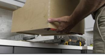
Press the clips under the trash organizer to release preinstalled slides, separating the organizer from the base.
