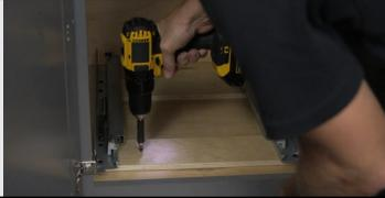
Secure the base unit by screwing through the plywood runners with 4 coarse-thread wood screws. #8 X 1" screws provided.
