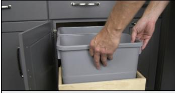
Slide the unit out of the cabinet. Insert the plastic trash bins into the pullout.
